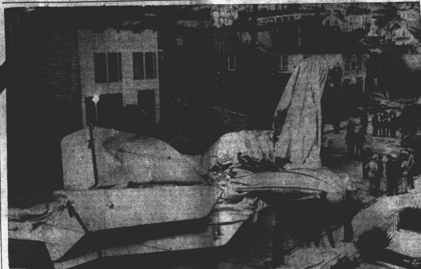
This Navy patrol blimp is shown sprawled in the street of a San Francisco suburb after it drifted across rooftops and crashed without its crew. The craft had been on routine submarine patrol and carried two officers as crewmen. Two lifebelts were missing and the Navy launched an intensive search of the waters off San Francisco. It drifted in with motors off and showed tears in its side before being further damaged in landing.
