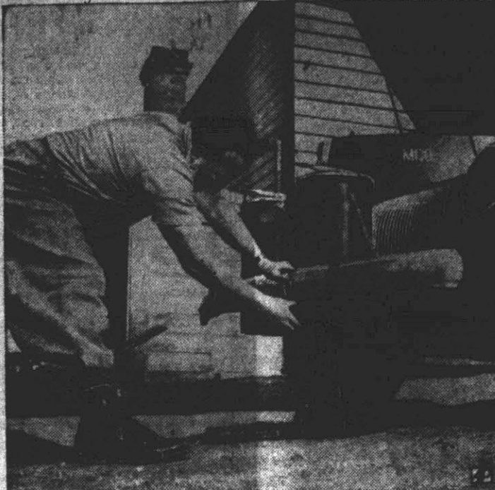
MESSY JOB—Draining the sludge out of the filter is one of life's minor annoyances for Australian motorists resorting to charcoal power for their vehicles in wartime. Here Morris Dowd demonstrates how it's done.
