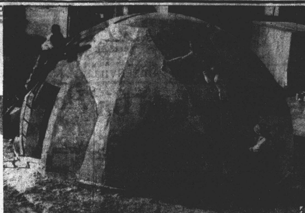
'DOME OF SAFETY' DOWN UNDER—Constructed of 66 tons of concrete, this "dome of safety" built for protection against possible air raids in Sydney, N.S.W., comfortably seated 60 persons during a test. Victor G. Steer, architect at Sydney Technical College, developed the shelter, using this design as affording greatest strength with use of least material.
