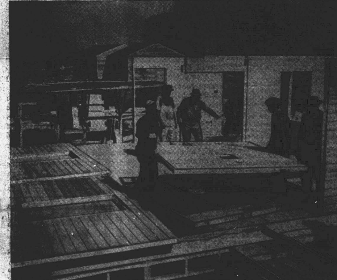
INSTALLING WALL PANELS —Workmen installing an interior wall panel in a structure of a war housing project at Hampton Roads, Va. Prefabrication is reported to be saving time.
