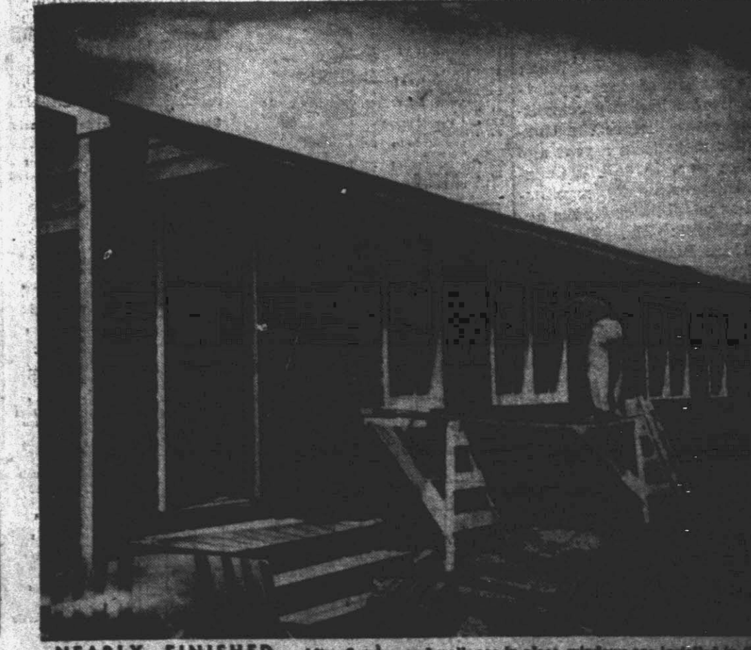
NEARLY FINISHED —After flooring and walls are in place, windows are installed in this prefabricated house in a war housing project under federal housing authority at Hampton Roads, Va.
