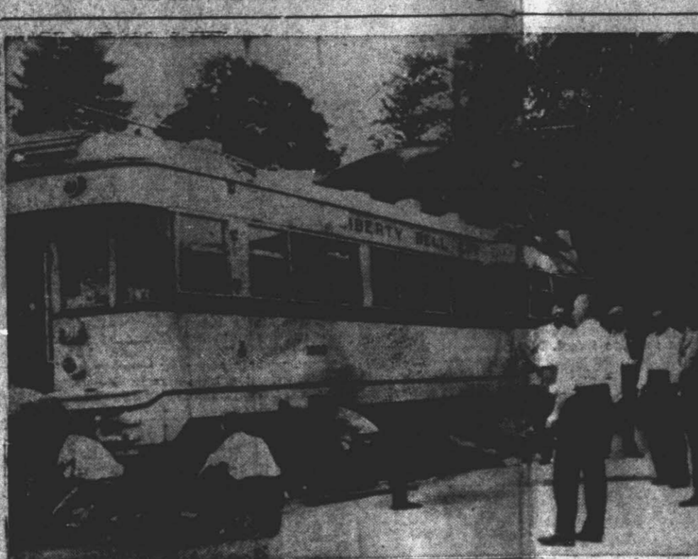
Workmen attempted to disassemble an interurban passenger trolley car and an express freight at Norristown, Pa., after a head-on collision that killed 10 persons and injured 22 others. The freight, running down grade, smashed through nearly a third of the passenger car.
