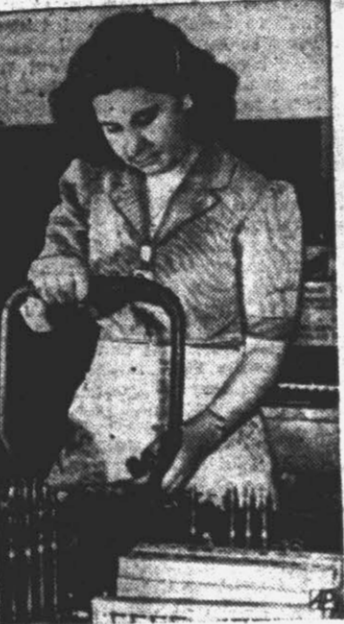
LOADING —Woman worker loads .50 calibre machine gun ammunition into metallic link belts at an army arsenal. Process requires single motion of U-shaped handle.
