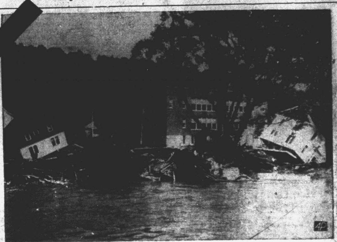
Subsiding flood water in Honesdale, Pa., a mountain resort town, left the wreckage of homes on the banks of the Lackawaxen river. At least 13 persons perished here. The total death toll for the entire eastern Pennsylvania flood area was at least 33. Scores were still missing. The Red Cross is feeding 3,000 homeless persons at Honesdale.
