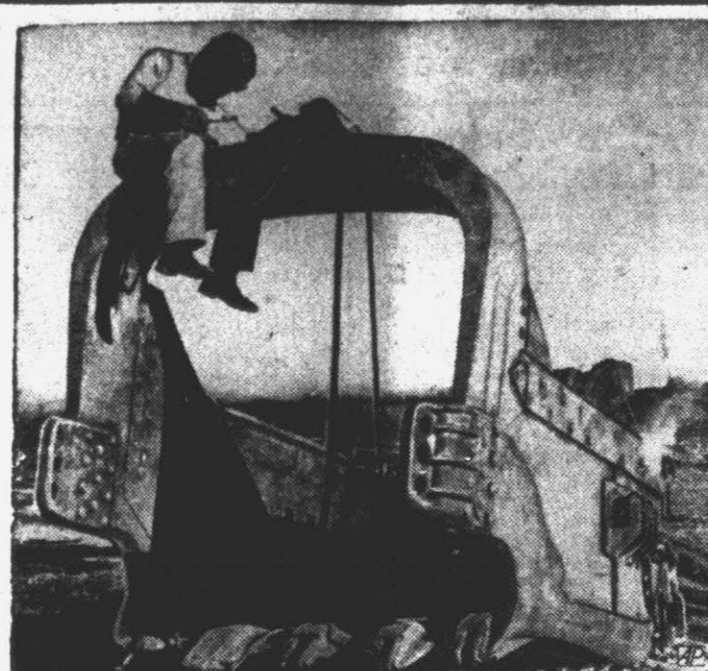
GROTESQUE DENTISTRY—Welder works on mighty jaw of excavating machine used on Shasta dam in California.
