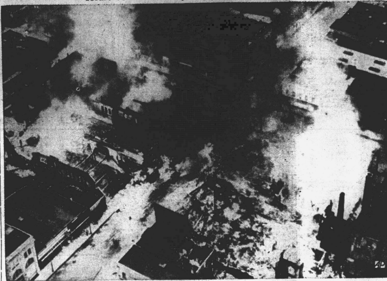
This mass of smoldering ruins was left by a fire that swept through the heart of Kewanee, Ill., and destroyed or damaged scores of buildings in the business district. Police Chief George Nelson said the damage might reach $2,000,000, including smoke and water damage. There were no known dead and only two firemen were hurt. The exact cause of the conflagration was not determined immediately.
