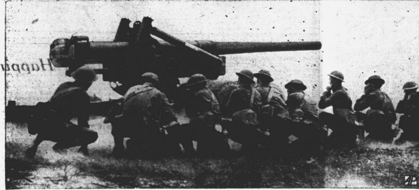
PICTURE WITH SOUND EFFECTS.—Army's longest range field piece, this 155 mm. rifle speaks out at Fort Bragg, N. C. Its range is 17 miles. The gun is drawn by 175 h.p. tractor, the gun and tractor together weighing 30 tons.
