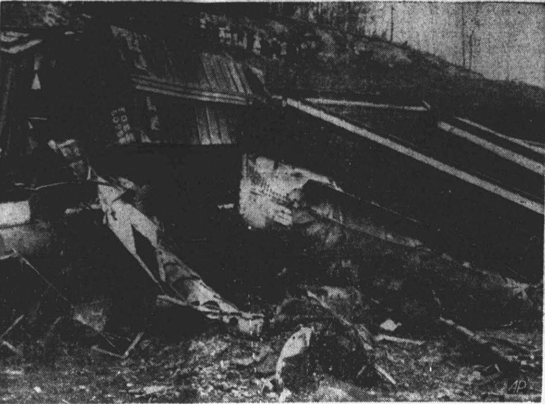
So strong was the force of a tornado that swept sections of the Mississippi valley and the middle west that it overturned this string of nine freight cars at Middlegrove, Ill. The storm left 20 dead, 170 injured and hundreds homeless in several areas of Illinois. Throughout the whole tornado area, at least 123 were killed and about 900 injured. In Mississippi 65 were killed and 630 injured. Tennessee's toll was at least 20 dead and 100 injured.
