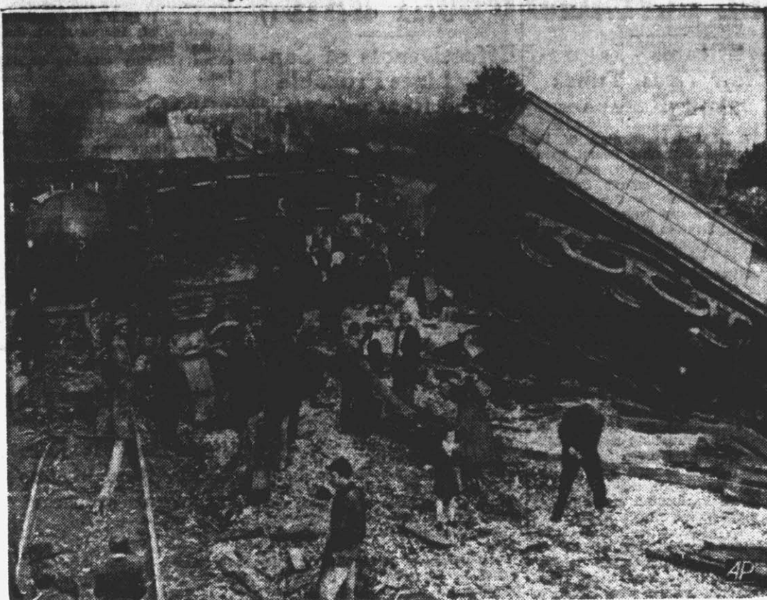
Wreckage litters the mainline of the Nashville, Chattanooga and St. Louis railroad near Chattanooga, Tenn., after derailment of the fast passenger train, Dixie Flyer, en route from Jacksonville, Fla., to Chicago. Engineer Ballentine and Fireman L. W. Arnold were killed, another trainman was injured seriously and six persons received slight injuries. In the distance is a freight train delayed by the wreck.
