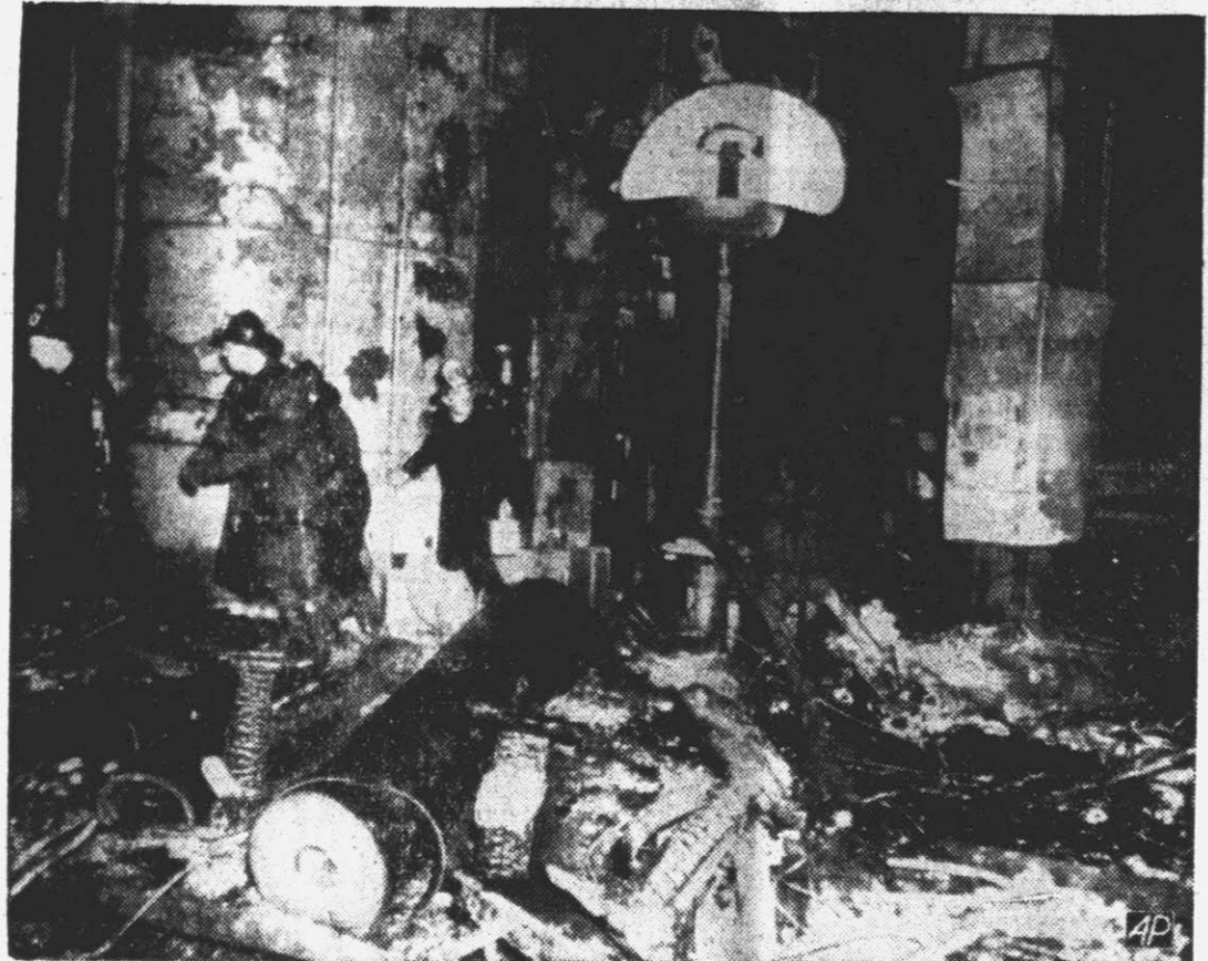
This was the scene in the grand ballroom of the once proud liner Normandie as firemen picked their way through the charred wreckage during the fire that swept the ship at her New York pier February 9 where workmen were converting her into an auxiliary vessel for use by the Navy as the U. S. S. LaFayette. This official U. S. Navy picture, released from Washington February 12, was made before the Normandie turned over.
