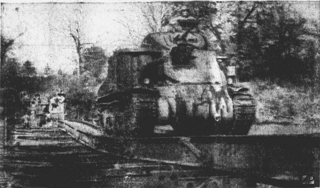
A new type of military bridge, in which rubberized fabric pontoons are used to support steel treadways, was demonstrated to army officials at Fort Benning, Ga., December 19 by the 17th Engineer Battalion of the Second Armored Division. Top: Soldiers maneuver the rubber pontoons into position in the Chattahoochee river. Bottom: Twenty-eight ton medium tanks roll across the bridge which was built in two hours and six minutes. Army men say the new span can be built four times as fast as the old type made of aluminum boats and wooden structures.
