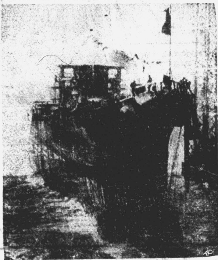
The 10,000 ton cruiser U. S. S. Columbia slides down the ways at the New York Shipbuilding Corporation yard at Camden, N. J., after being christened by Miss Jean Adams Paschal of Columbia, S. C., the city for which the vessel was named. The ship will be commissioned for service next year.
