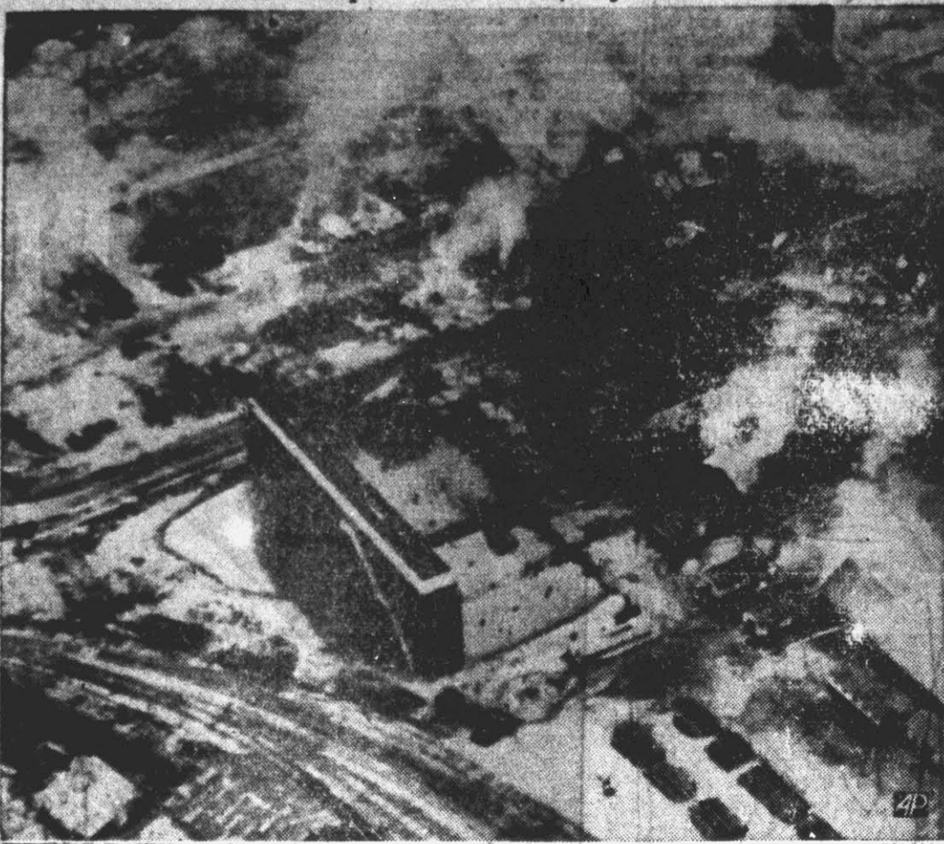
This scene of smoking ruins was left by an explosion and fire which killed three persons and injured 17 others at the Phillips Petroleum company at Okmulgee, Okla. Two stills exploded and started the fire which swept through the gasoline department of the plant.
