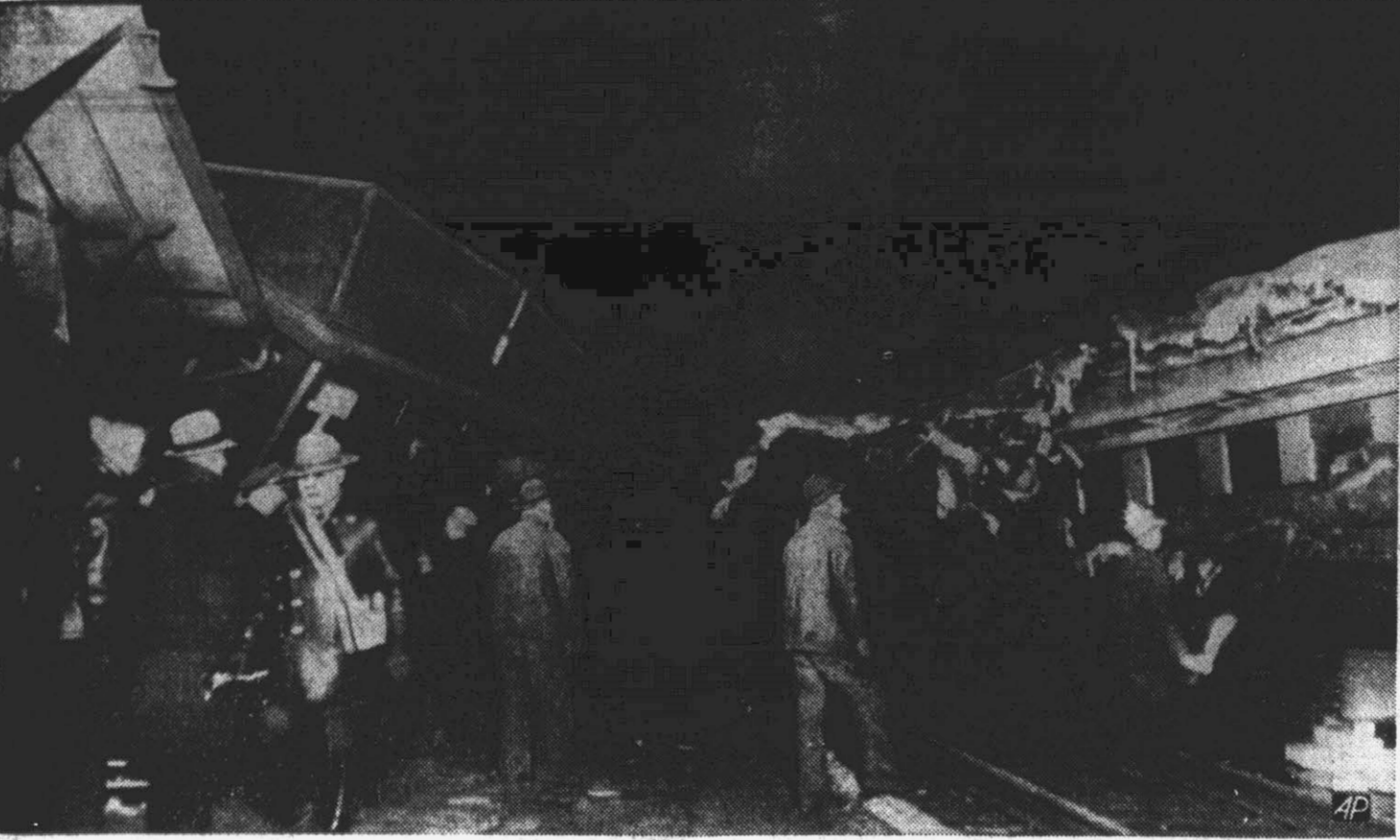
Eleven persons were killed and about 50 were injured in this mass of wreckage of the Pennsylvania railroad's fast passenger train, "The Pennsylvania," near Dunkirk, Ohio. The overturned locomotive lies against twisted debris of a signal tower (left). Back of the engine is one of the eight wrecked cars. It was derailed by a cylinder head blown off the locomotive of a freight train passing in the opposite direction.
