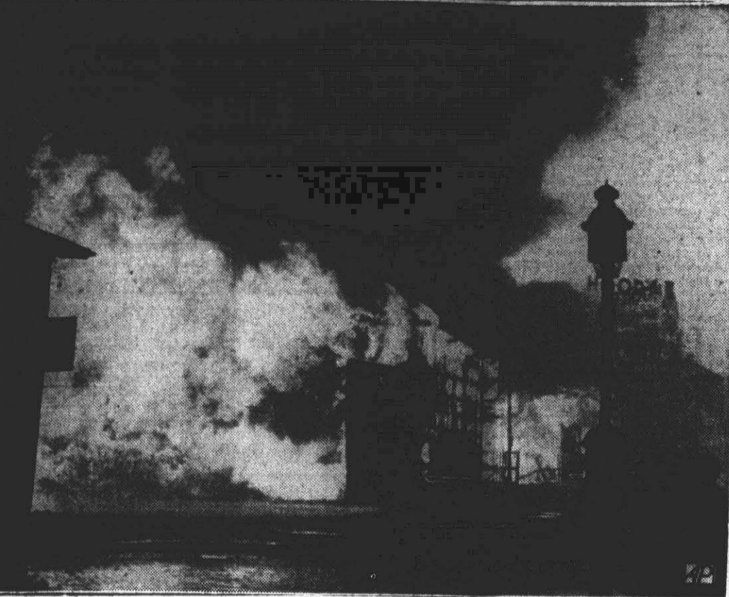
Raging flames eat their way through a building during a fire that swept through four huge warehouses in the freight yards of the Boston and Maine railroad in the Charlestown section of Boston. Damage was estimated at more than $1,000,000. At the right is the box from which the first alarm was turned in.
