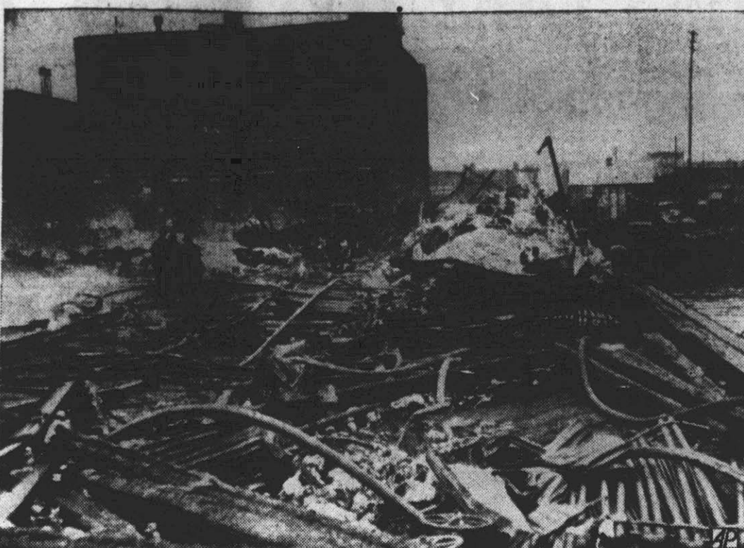
Twisted steel girders and charred debris litter the Brooklyn, N. Y., pier after the raging waterfront fire which also destroyed the Cub a Mail Line freighter Panuco, numerous smaller craft and left at least seven persons dead in its wake. Damage was estimated at approximately $1,500,000.
