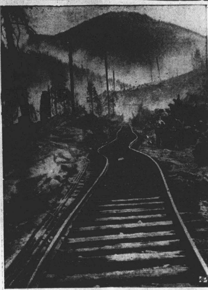
FURY OF THE FLAMES —So hot was the forest fire that swept through parts of the Snohomish national forest in the state of Washington that the heat twisted these railroad tracks. Some 500 men were called to fight the 6,500-acre blaze.
