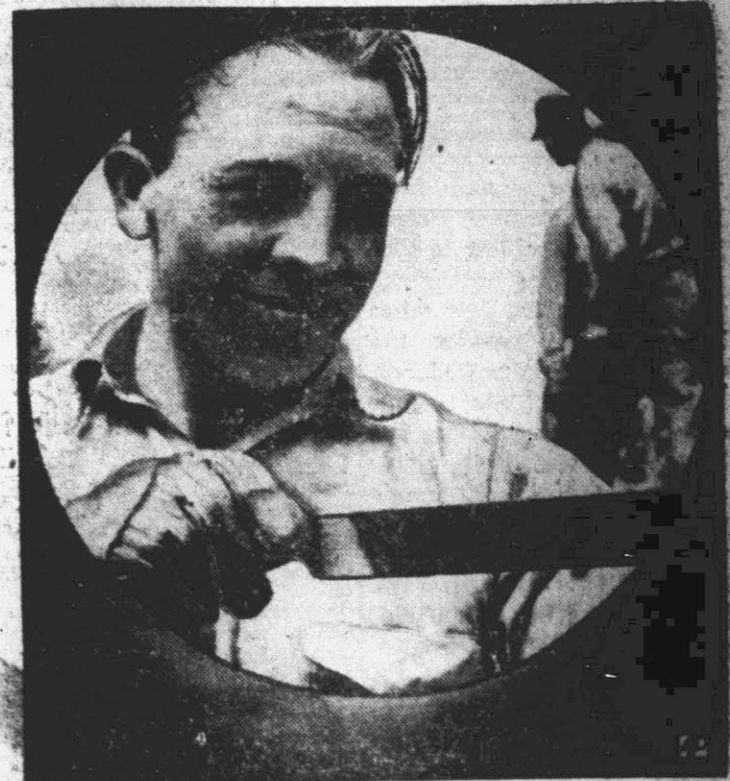
INSIDE STUFF —Intently a workman files the end of 12 3/4-inch pipe, before welding, on the $8,000,000 Portland, Me., to Montreal oil pipe line being built. Overland pipe route will save tankers' 12 days' passage in the St. Lawrence.
