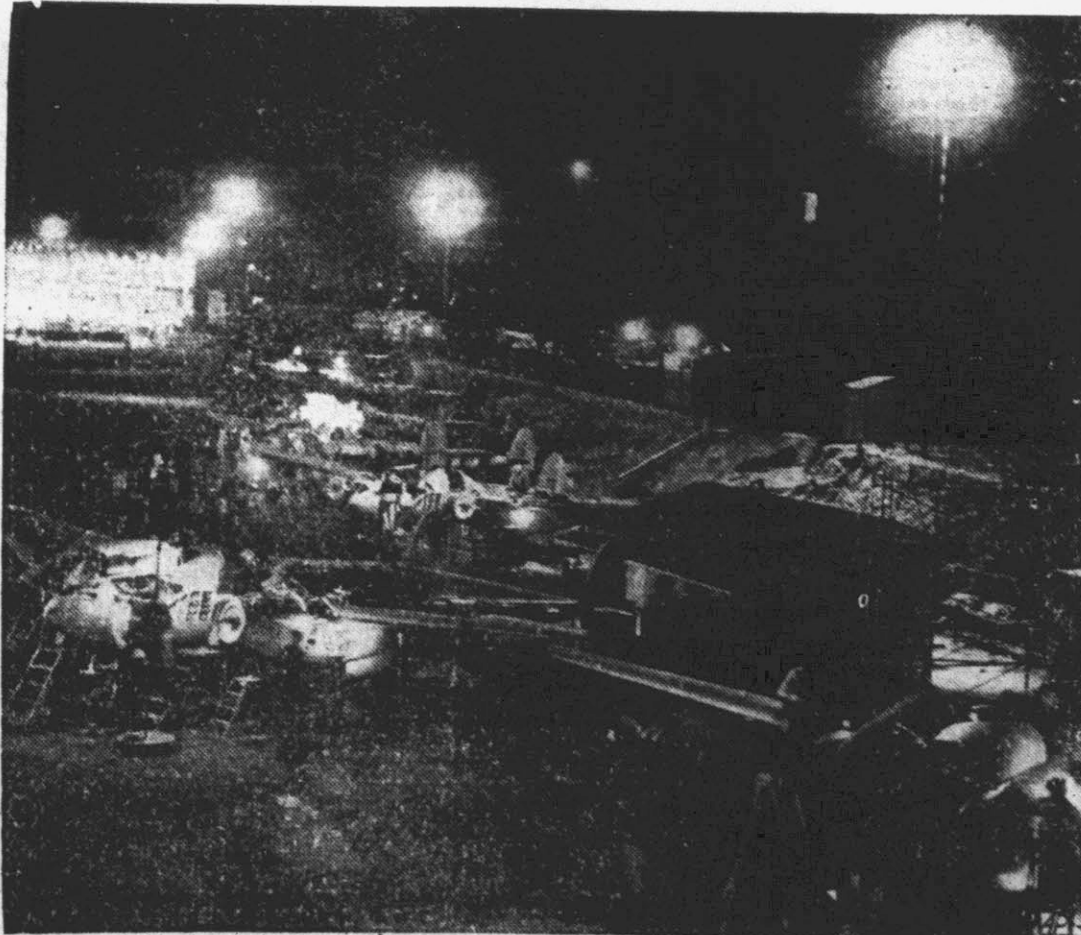
STARLIGHT ASSEMBLY —The final assembly of Lockheed P-38 pursuit planes at the Burbank, Calif., plant goes on outdoors under floodlights, because of lack of room inside the plant.
