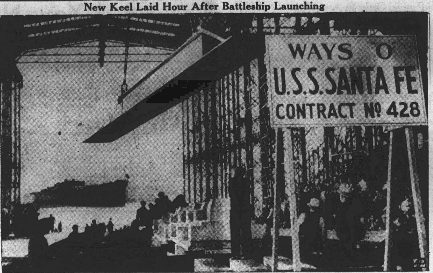
With the ways still warm from the launching of the 35,000-ton battleship South Dakota (background), the keel was swung into place for the 10,000-ton cruiser Santa Fe which will be built on the same ways. The scene is the yards of the New York Shipbuilding Corporation in Camden, N. J.
