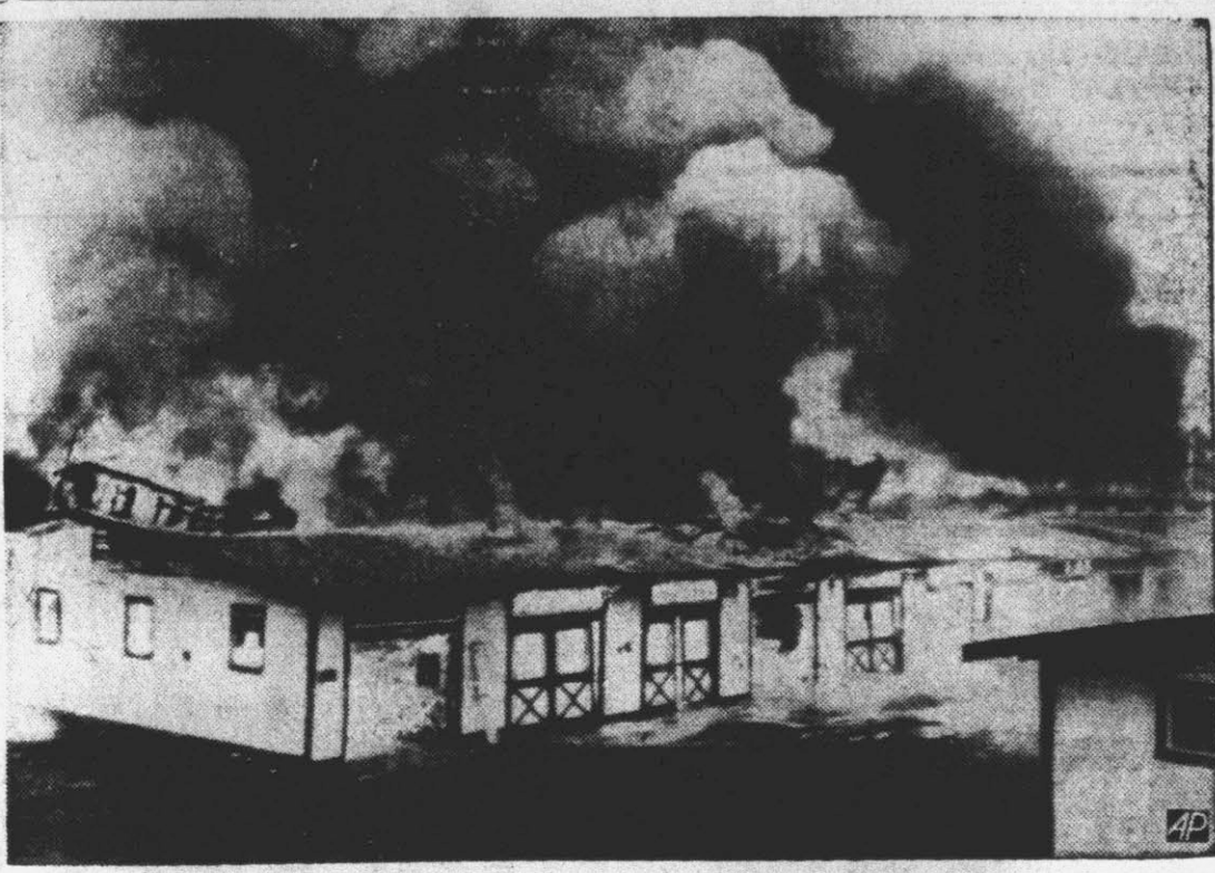
Flames destroyed 30 garages and one racing car at the Indianapolis Motor Speedway shortly before the start of the 29th annual 500-mile Memorial Day race. This picture was made at the peak of the fire. Eddie Offutt, owner of the destroyed car, said the flames started from spilled gasoline accidentally ignited by static electricity or a match.
