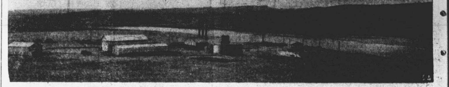
Modern oil pumping station on a pipeline which stretches across barren, eroded Iraq.
