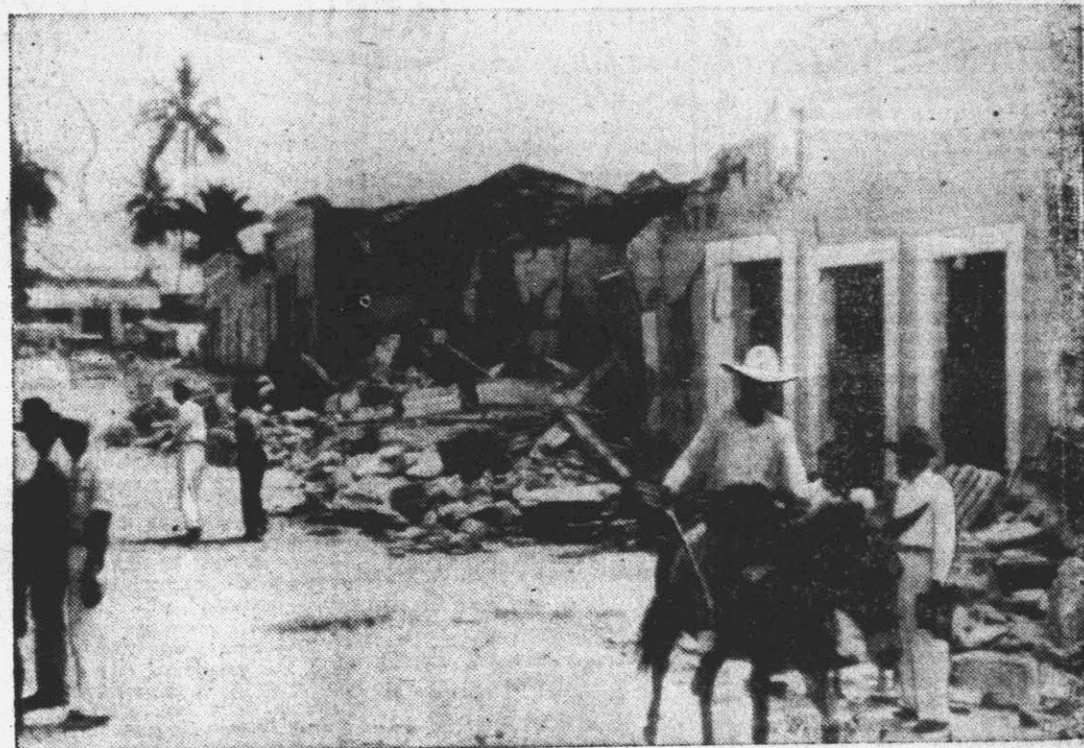
This street of shattered stores and homes was left in the wake of the earthquake that brought death and devastation to the city of Colima, Mexico. Now that the terror of the quake has passed, residents seem to be taking it calmly, as indicated by the man on the slow-moving burro and men talking in the street.
