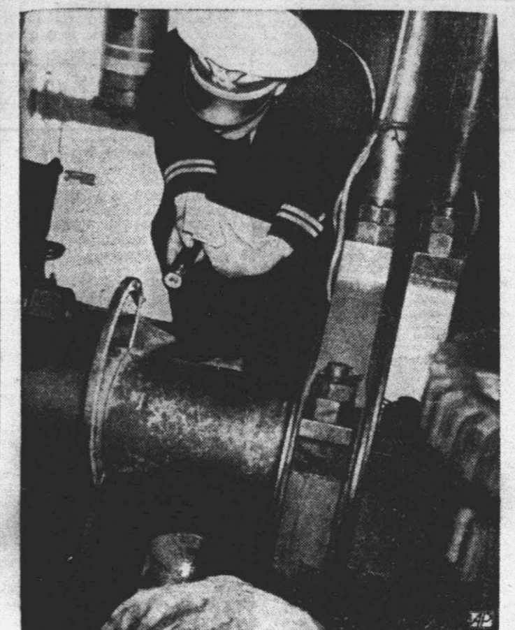
When Coast Guardsmen seized the Italian freighter Ada O. in New Orleans harbor under government orders, they found the 14-inch propeller shaft sawed almost in two. Coast Guard Lieut. E. J. Roland inspects the damaged shaft with the hacksaw still embedded. The freighter was among more than 60 Italian, German and Danish vessels taken into custody by the Coast Guard in United States ports because some crew members were sabotaging their own ships.
