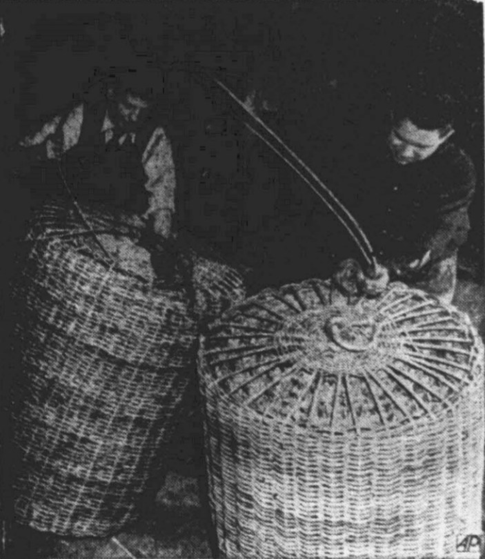
WEAVING FOR WARSHIPS —Hands of Jake Turose (left) and Valentine Kruk that once wove baby bassinets now build bumpers for U. S. warships—fenders woven of rattan with a forging iron as a center piece. The bumpers, dangled over ship-side, prevent damage from piers or other vessels. Turose and Kruk learned their trade as youngsters in Poland.
