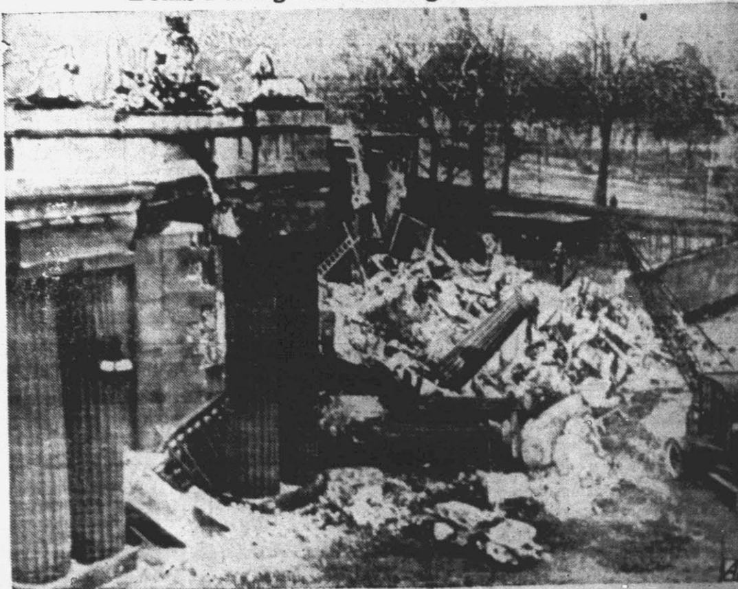
Three high explosive air raid bombs did this damage at a Buckingham Palace lodge in London recently, wrecking the lodge house and part of the pillars of the portico at the left. Royal insignia still surmounts pillars. A policeman was killed during the raid.
