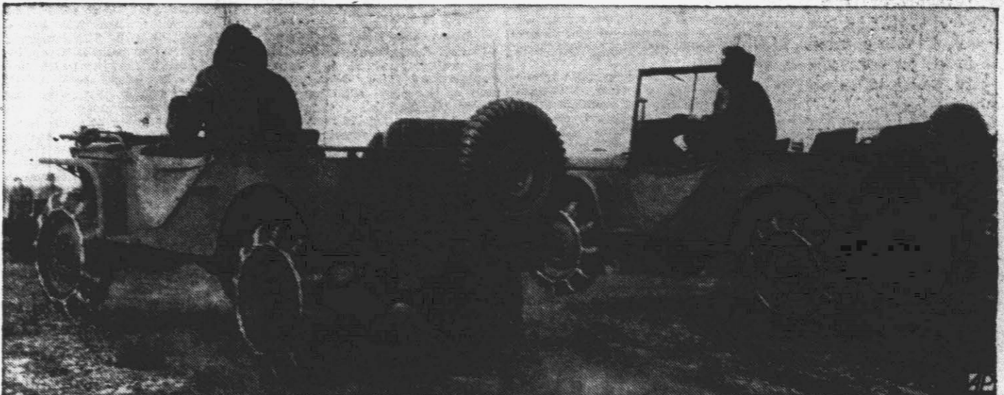
ROUGH AND READY BUT MOSTLY ROUGH—Two of the new "blitz buggies" being built by Henry Ford bounce along at Detroit. They're U. S. army scout cars, with overall length of 127 1/2 inches, and speed of 57 m.p.h. Other features: blackout lamps front and rear; hand grips on outside enabling crew to lift machine; straps and railings inside car for safety in rough cross-country riding. Car is small enough to be concealed in a field in quantities and light enough (2,100 lbs.) to be carried in a bomber.
