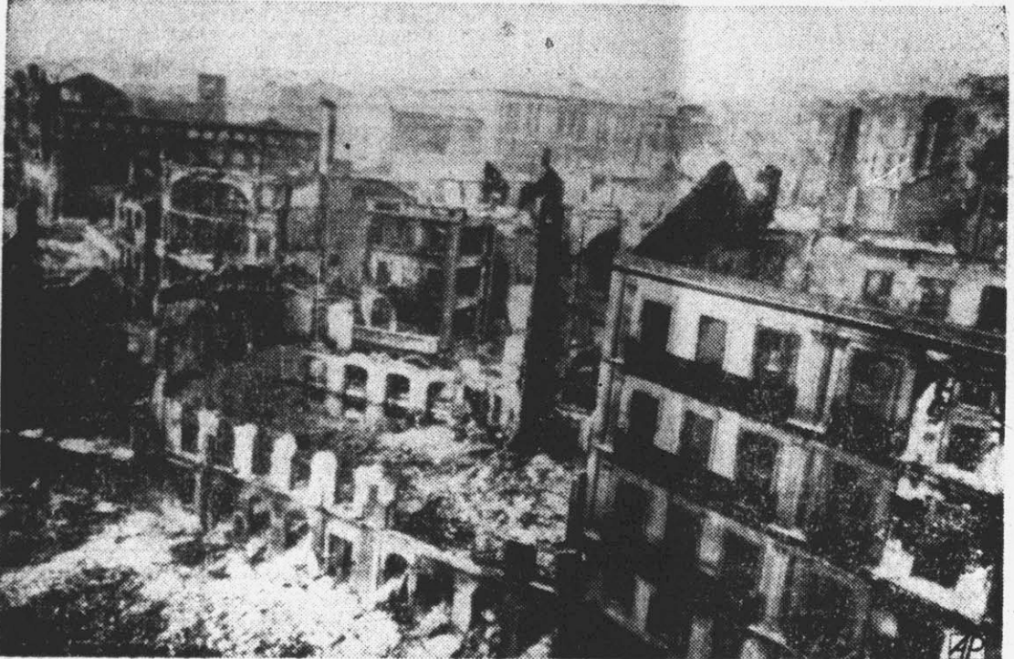
This mass of ruins was left in the wake of a gale-driven fire that swept over the Spanish port city of Santander. At least 26 persons were killed and more than 200 homes were destroyed by the flames and the storm.
