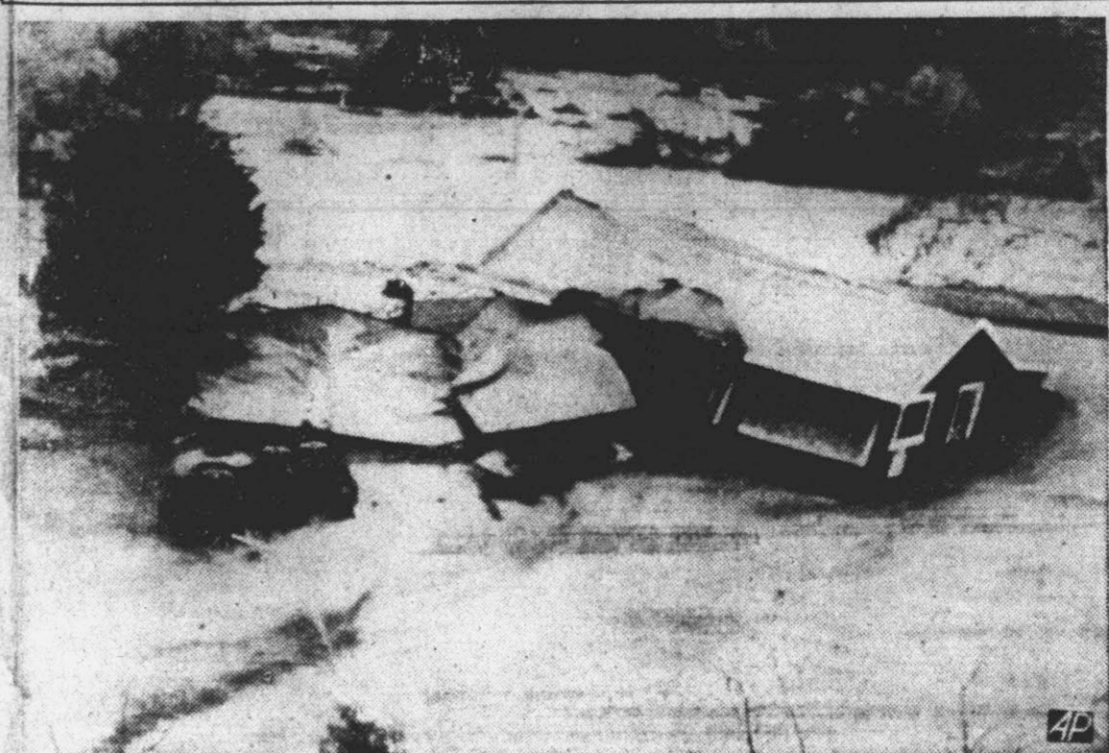
Torrents of water, gushing through Topanga canyon near Los Angeles, undermined this house and toppled it into the stream during a flood resulting from heavy rain that swept most of southern California. Two deaths were indirectly attributed to the deluge.
