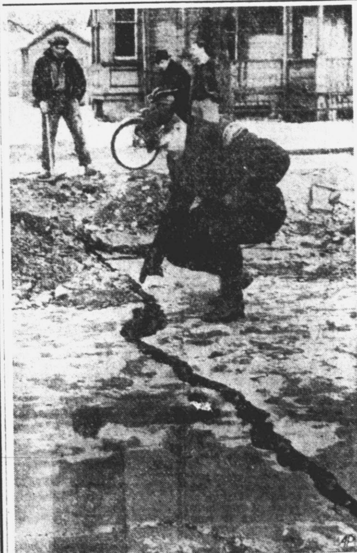
STREET SEAM —When part of West Pittston, Pa., a town of 8,000, settled recently due to underlinings of mines in that area, this fissure appeared in street. Another Pennsylvania anthracite town, Shenandoah, was similarly affected last year.
