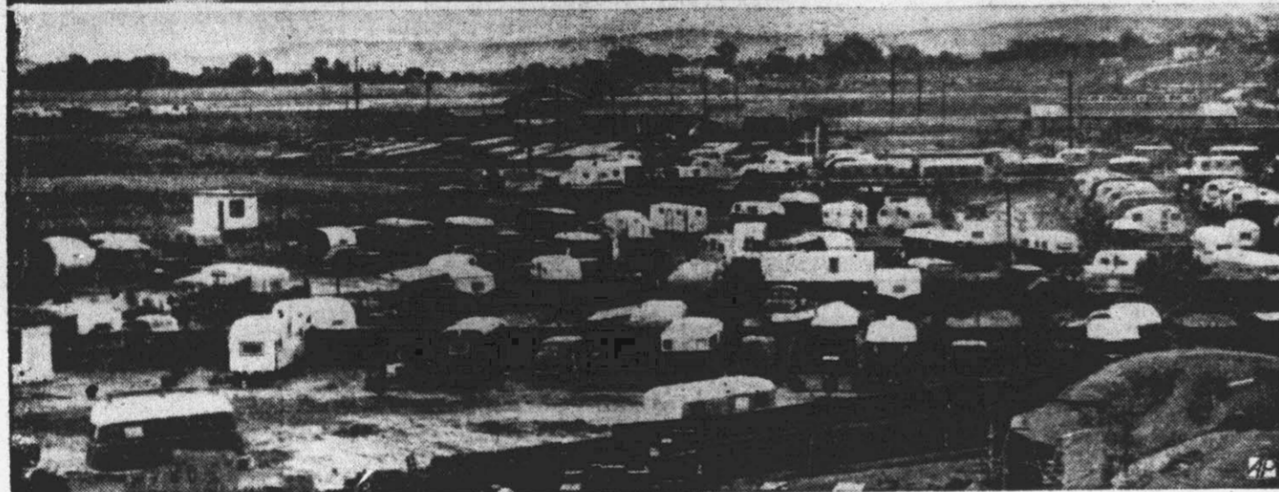
BOOM'S ON, AND WE DON'T MEAN CANNON —California, like other states where defense activity is rushing, has a building boom on its hands, especially in those sections where quarters for the soldiers are being constructed. Here are scenes from San Diego: additional naval facilities and a coast artillery corps replacement center to house 8,500 men are being built there. In upper view is the barracks being built at Camp Callan near San Diego. Below is a trailer colony for workmen unable to find homes.
