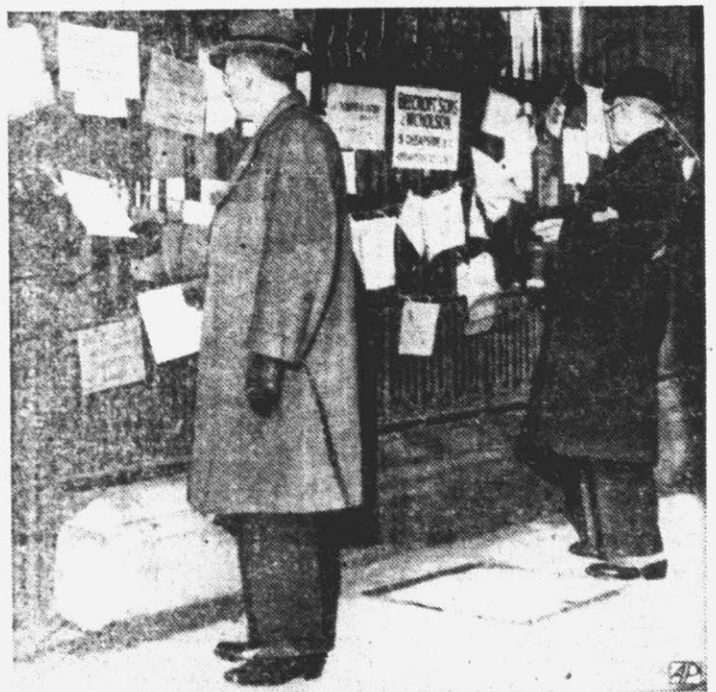
'BLITZ' DIRECTORY —To help their clients find them, bombed-out firms in "The City," London, put their addresses on this fence railing which is now a virtual "blitz" directory.
