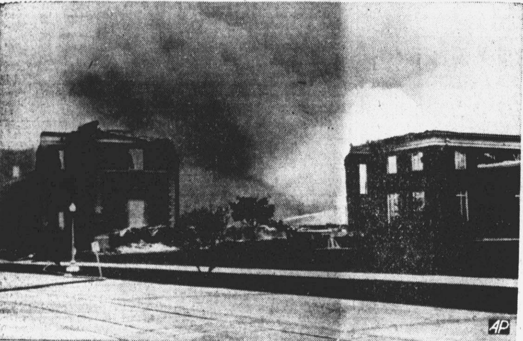
Fire of undetermined origin did damage estimated at $275,000 at the United States naval base in Norfolk, Va. The building with the center section caved in was the administration building in which a quantity of official records and documents was destroyed. Smoke pours out of the runs. A board of inquiry is investigating.
