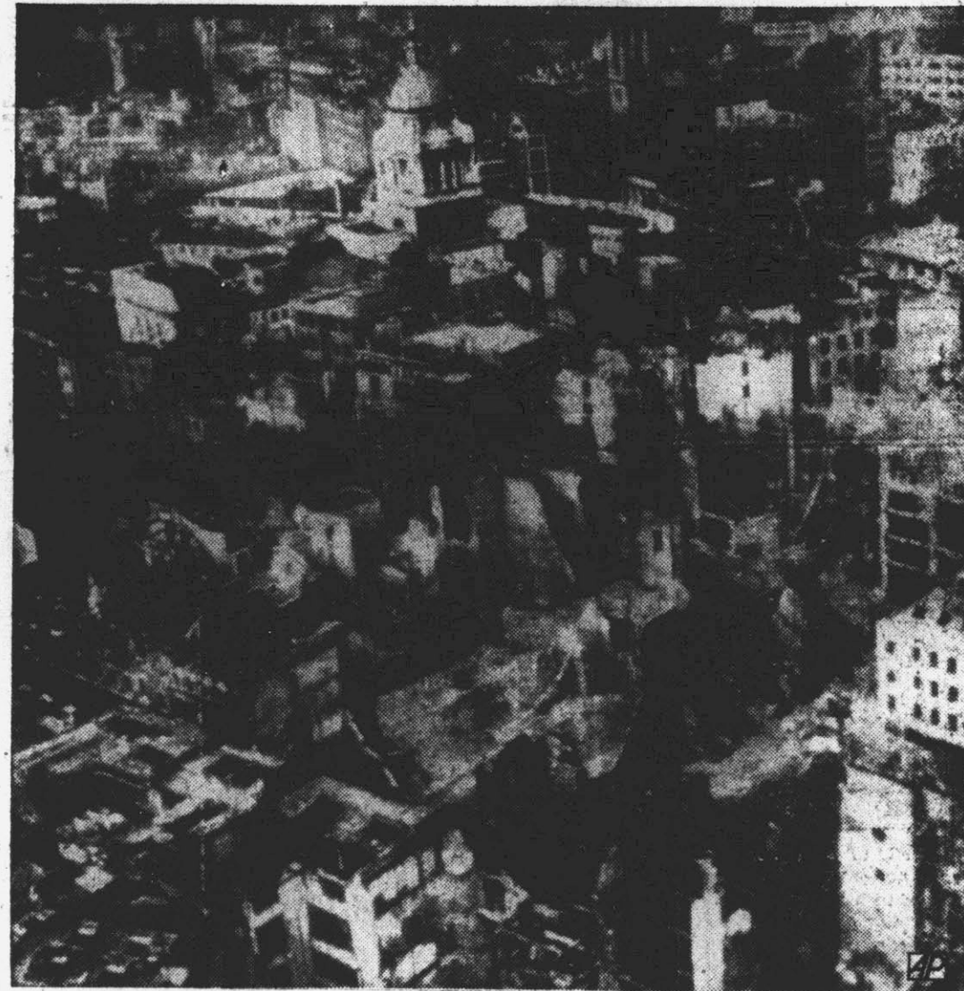
The area in and around Paternoster Row in the ancient "city" of London presented this scene of damaged buildings after German air raiders laid down a deluge of fire bombs December 29. The dome in the background is that of Old Bailey. This picture came from London by radio.
