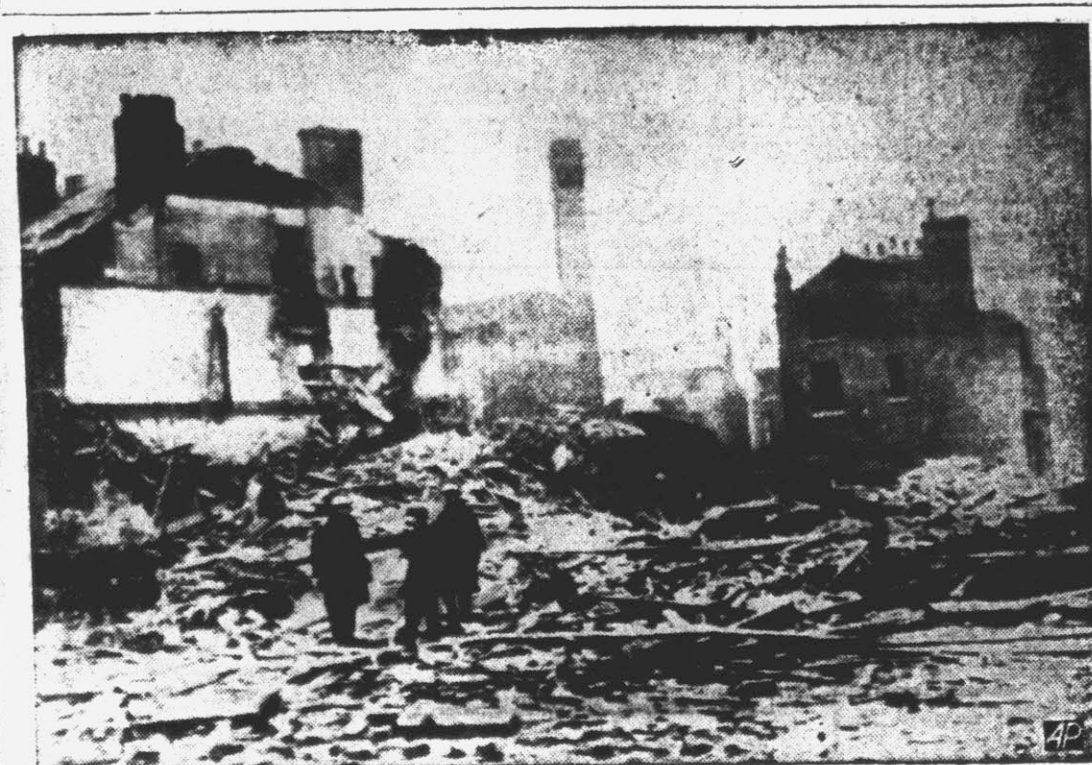
Air raid wardens inspect the ruins of houses demolished during a German air raid on Manchester, England, in the industrial heart of the British Isles. (This picture by radio from London).
