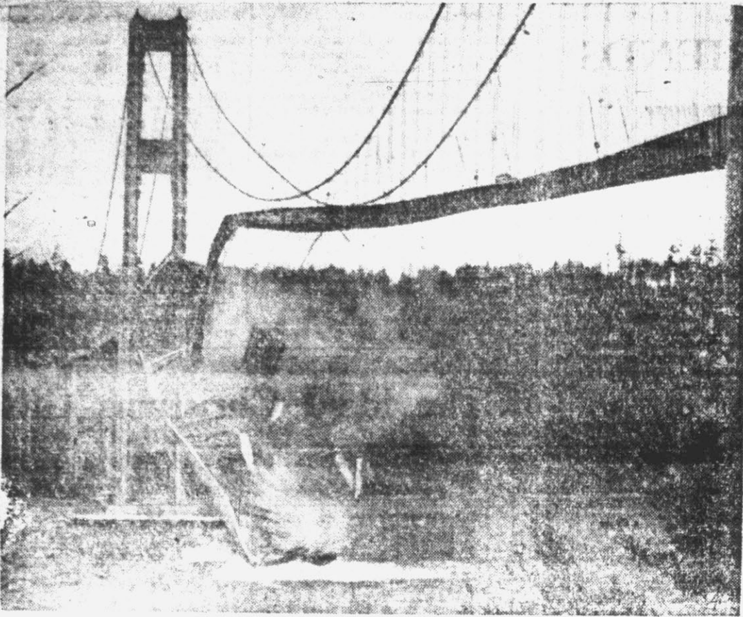
'GALLOPING GERTIE' GOES Wind-blamed crackup of 2,800-foot center span of the new $8,400,000 Narrows bridge at Tacoma, Wash.—third longest single suspension in world—put an end Nov. 7 to the shimmying undulations that gave the bridge its nickname, "Galloping Gertie." Nature's fury in 1940 was also responsible for earthquakes in Turkey (January); Peru (May); Romania (November).
