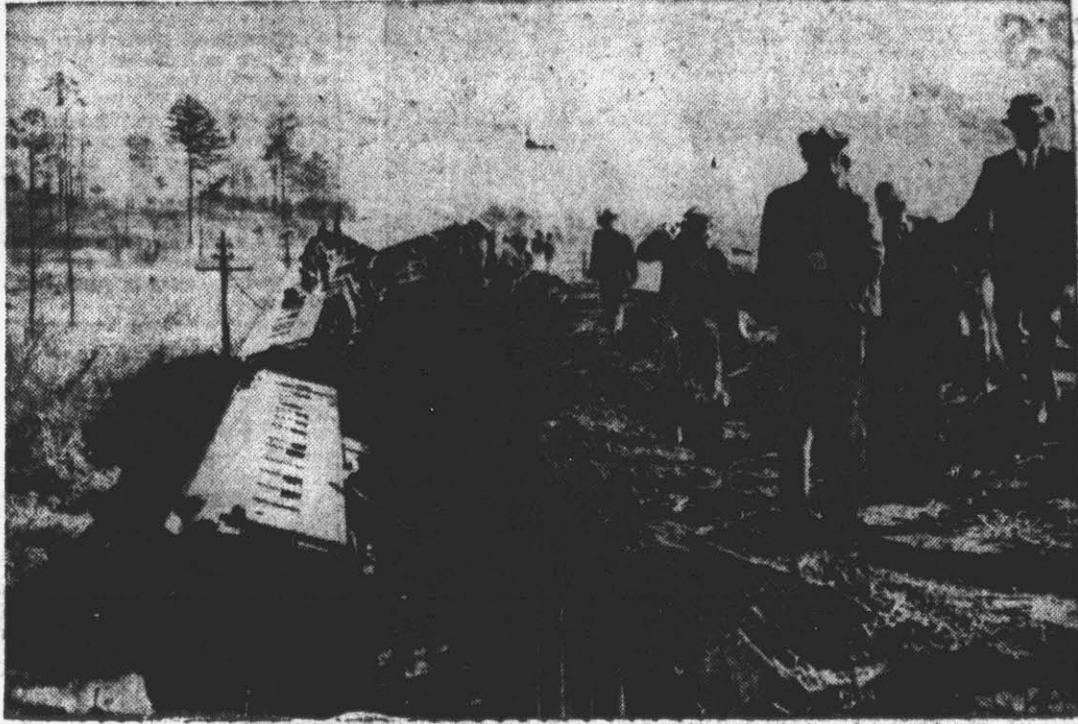
At least seven persons, including E. E. Norris, president of the Southern Railway System, were injured in the derailment of the Southern's fast passenger train, "The Ponce de Leon," 14 miles south of Atlanta. Three cars overturned near the end of this trestle and others left the rails but remained upright. President Norris was riding in his private car (foreground). The train was en route from Chicago to Florida.
