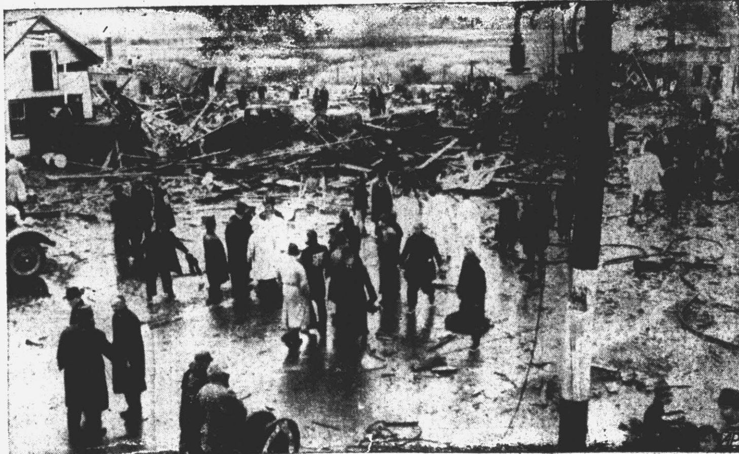
At least five persons were killed and the factory of the United Railway Signal Corporation at Woodbridge, N. J., was wrecked by a terrific explosion that jarred the countryside for miles around. Only a portion of one of the 15 buildings in the plant remained standing. Firemen, rescue workers and spectators are viewing the wreckage.
