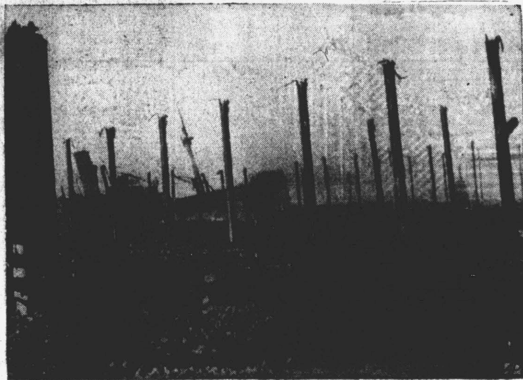
British sources describe this cablephoto as a view of a Thames river dock shed wrecked by German air raids on London over the week-end. Only the upright steel framework remains to outline the ruins of the building. At the left is another building damaged by fire and in the background is a listing ship. British observers admitted the raids disrupted activity on London's docks. They said incoming food and supplies obviously will have to divert to other ports and be brought to London by trains and trucks.
