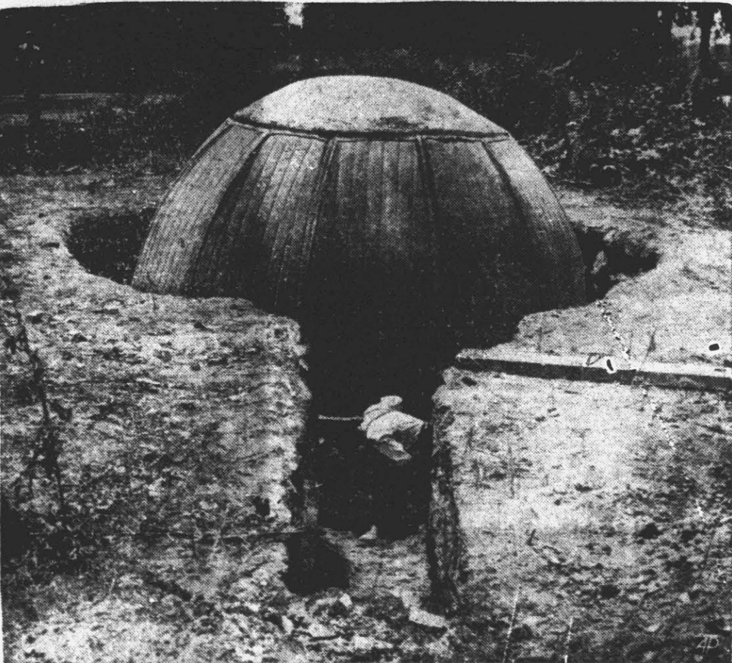
BITTER PILL—FOR AN ENEMY—At least one "John Public" inspects first-hand a bomb-resisting pillbox demonstrated to army and navy leaders in Washington at an isolated spot along the Potomac. Built of concrete in five hours, complete with gun opening and trench approach, the pillbox supported weight of three men a few hours later.
