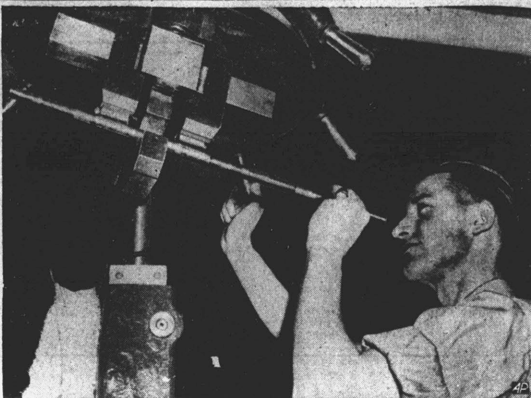
IT'S THE STRAIGHT GOODS—Most important is the job of Maurice J. Healey (above) at the U. S. armory in Springfield, Mass. He has to see that the rifle barrel is straight, a procedure called line straightening bore of barrel. The arsenal has set its production goal at 1,000 Garand semi-automatic rifles a day, in order to equip the expanding U. S. army.
