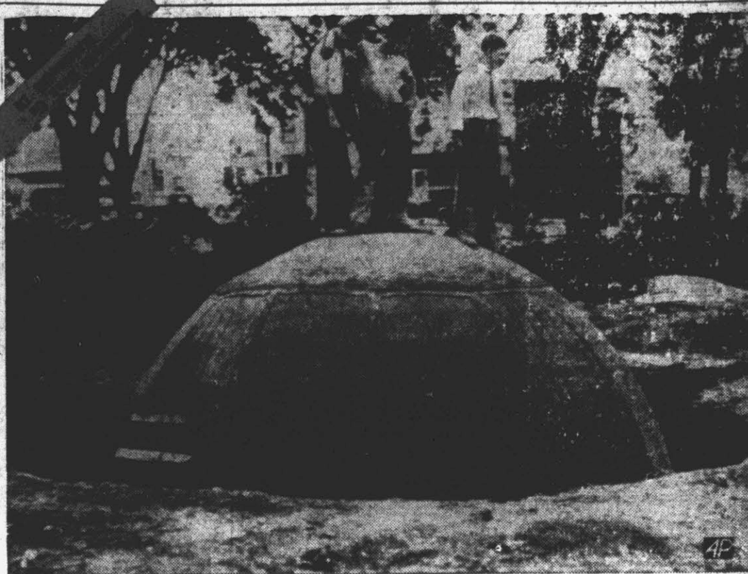
These concrete forts—demonstrated to Army and Navy leaders in Washington—are capable of springing up in a mushroom and looking the part as well. The forts are built of concrete in five hours, complete with gun openings and trench approach. The box was strong enough in a few hours to support the weight of the three men shown atop.
