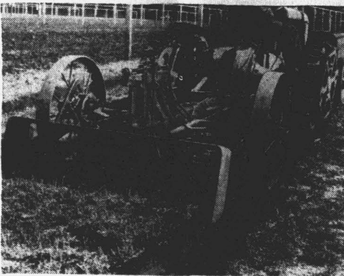
This harvesting machine digs up the plant, root and all, and chops it up preparatory to crushing in the pebble mill.
