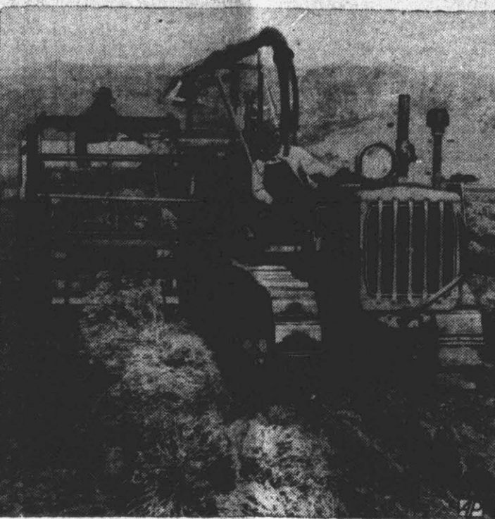
A subterranean knife dislodges guayule seedlings from their nursery bed preparatory to transplanting in the field.
