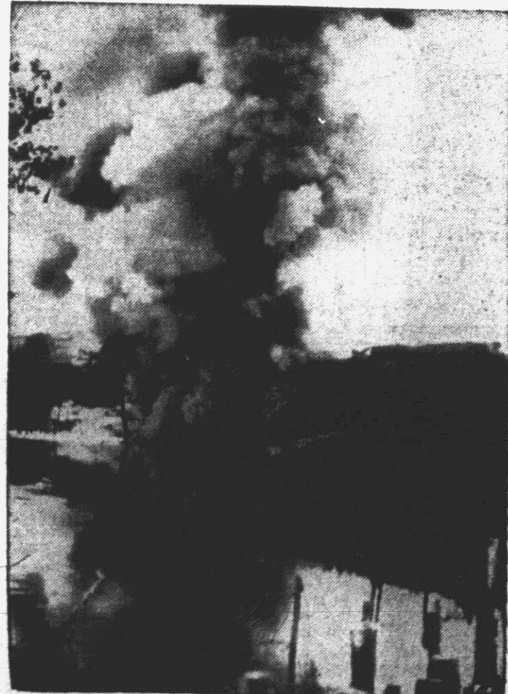
The French caption says this shows an explosion set off by the Allies to destroy a bridge in the path of advancing German troops somewhere in France. Note the wire entanglement in the foreground. Destruction of bridges was anticipated by the Germans who carry portable bridges, many of which had been "made to measure" to replace the ones destroyed.
