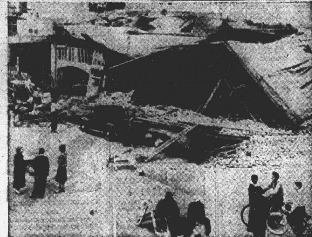
Here's a view of the main street in the town of Imperial, Calif., after an earthquake shook the entire Imperial Valley, killing eight persons, injuring more than 100 and doing damage estimated at $2,500,000.
