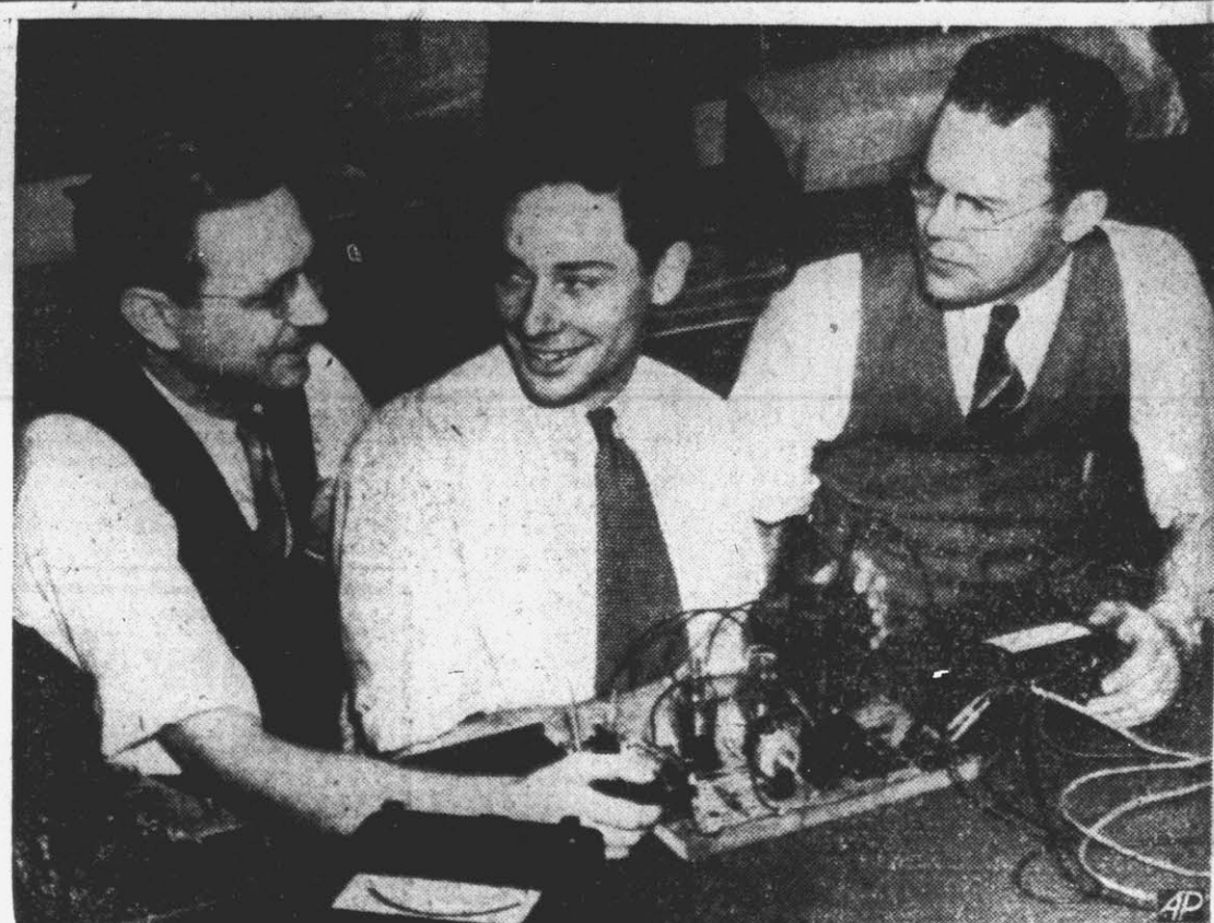
These Associated Press engineers, Charles W. Hubley, James C. Barnes and Alfred S. Gano (left to right), are shown in the AP laboratory in New York with the new amplifier-recifier — in effect, an "electrical lens"—They have built for wire-photo reception equipment. The device further improves the fidelity with which details of pictures sent by wire-photo are recorded on films.
