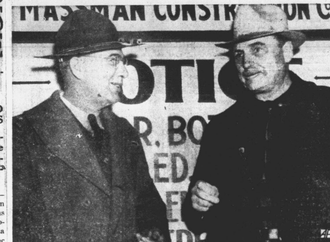
Maj. H. B. Parris (left) of the Oklahoma National Guard is shown with Construction Superintendent I. N. Towne at the Grand River dam near Disney, Okla., after Gov. Leon Phillips placed the dam under martial law in his "state's rights war" with the Federal Works Administration. The governor ordered the troops to prevent the dam from being completed unless the WPA pays $850,000 damages for roads and bridges that would be inundated by the dam.
