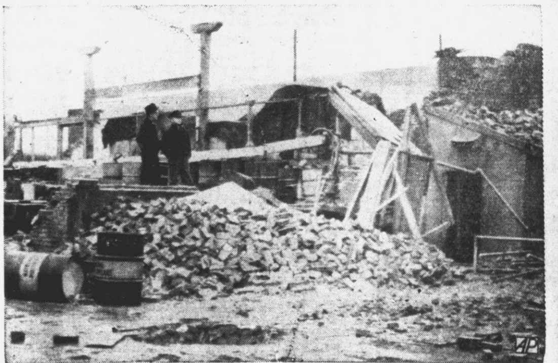
One child was killed, about 12 persons were injured and some 340 buildings were damaged by a tornado that struck Evansville, Ind. This picture shows all that remained of a National Refining company warehouse, one of numerous buildings demolished.
